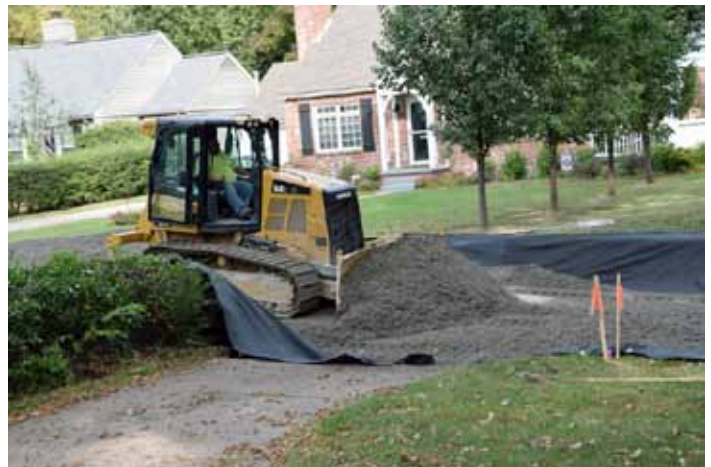
Gravel replaces dirt followed by new curbing and paving.
